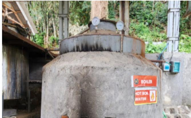
**Gambar 5. Pemasangan Pressure Gauge**
